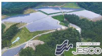
Mega Solar Panels in Japan built by JESCO.
